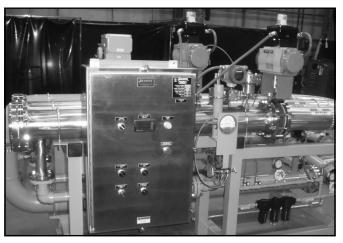
Figure 4.2. Air Flow Control Train
