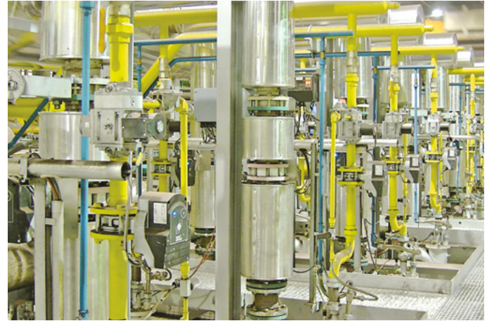
Walking beam furnace with overhead firing
